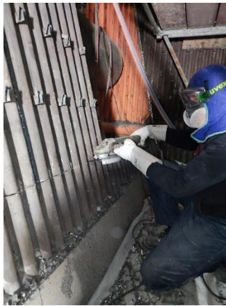
The cutting process with a large, heavy angle grinder in an awkward physical posture
